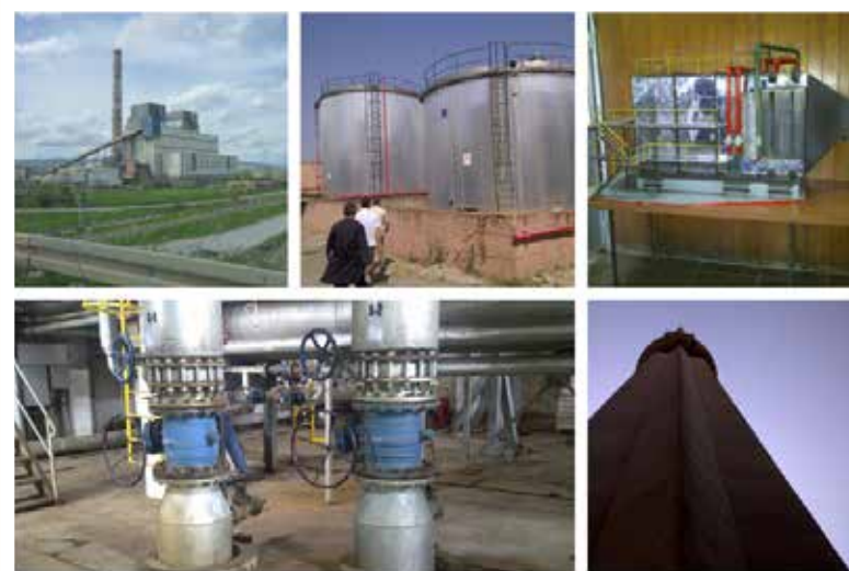
Figure 8: CHP plant in Pristina
