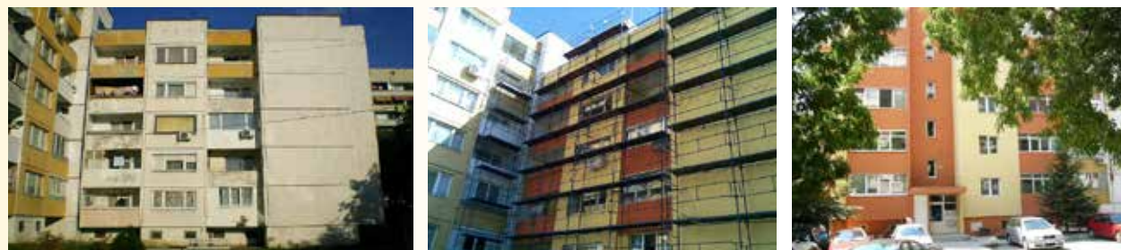
Figure 7: Demo renovation of residential multi-storey buildings in Bulgaria
