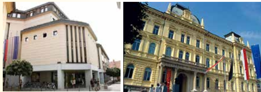
Figure 10: ESCO-serviced buildings in Maribor
